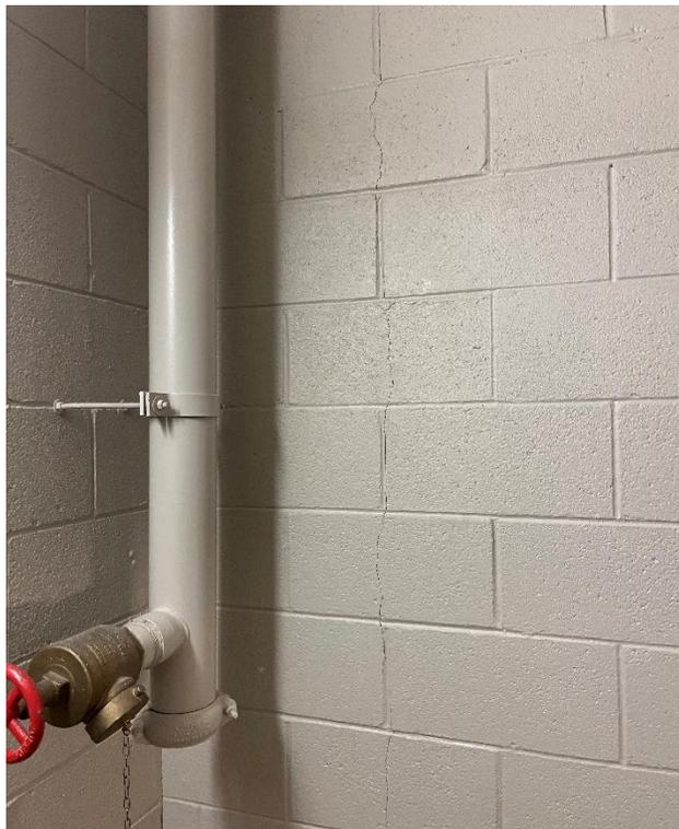
**Gum Spring Photograph 2 – Vertical Crack in Stair Shaft**
