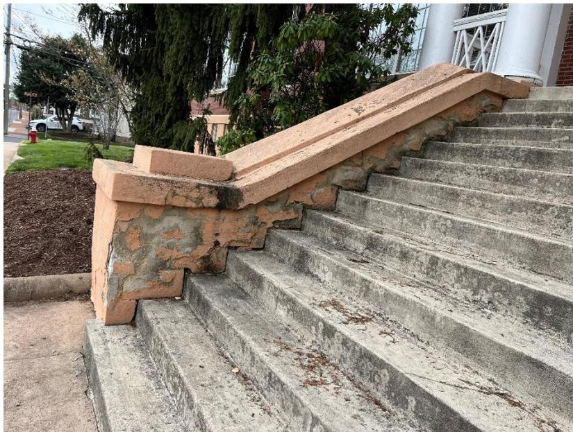
**Administration** Photograph 2 – Side Rail Separation / Spalling
