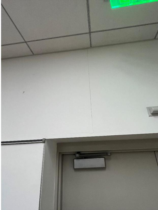
**Sterling** Photograph 3 – Crack in Interior Finishes
