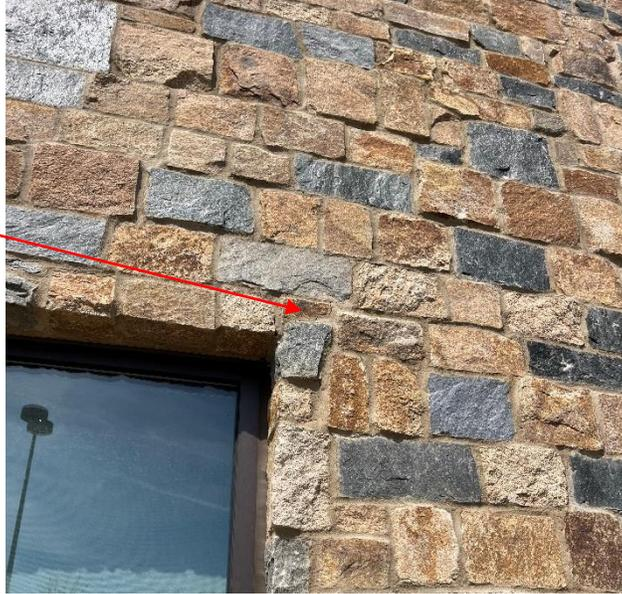
**Brambleton** Photograph 1 – Diagonal Crack in Stone Veneer
