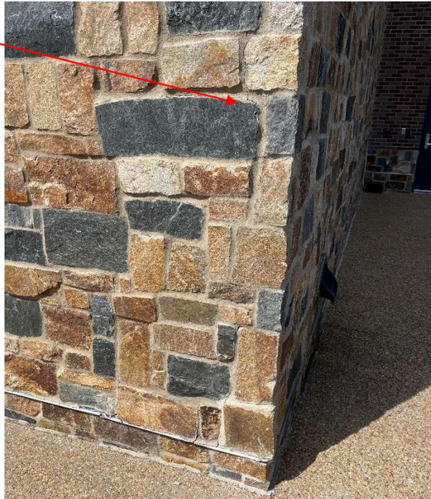
**Brambleton** Photograph 2 - Vertical Crack in Stone Veneer
