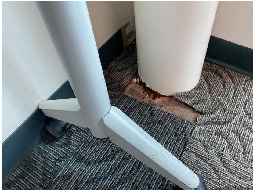
**Ashburn** Photograph 2 – Interior Column Corrosion at Base
