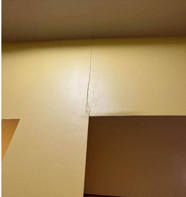
**Gum Spring Photograph 1 – Crack in Interior Finishes**
