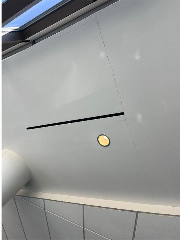
**Brambleton** Photograph 3 – Crack in Interior Finishes
