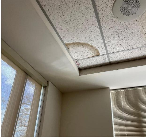
**Cascades** Photograph 5 – Moisture Damage at Ceiling Tiles
