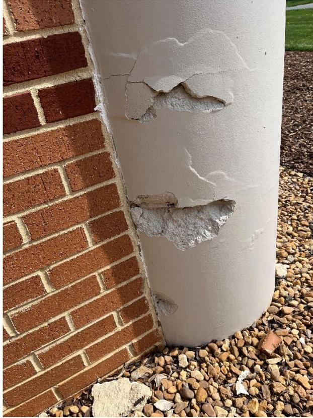
**Rust** Photograph 1 – Damaged Concrete at Column
