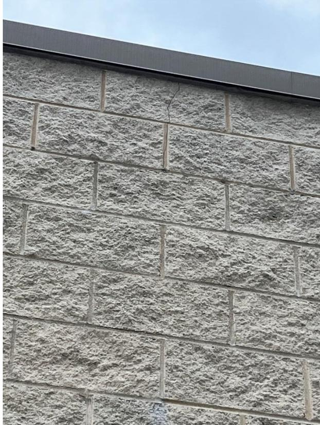
**Ashburn** Photograph 3 – Crack in Exterior Masonry
