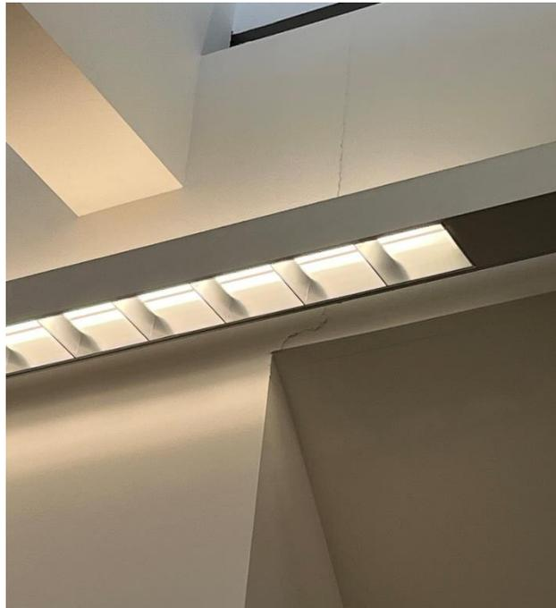
**Cascades** Photograph 4 – Typical Cracking of Interior Finishes
