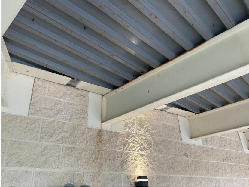
**Ashburn** Photograph 1 – Exterior Steel Corrosion
